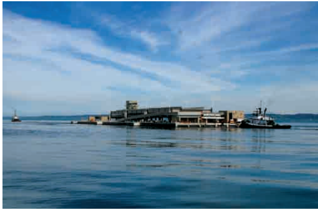
The Sidney Foss , in the lead, and the Shelley Foss move the east draw span of the Hood Canal Bridge up Puget Sound near the north end of Bainbridge Island on May 17. The tow measured 600 feet long, weighed 51,100 tons and drew 31.5 feet. Because of its bulk the tugs couldn't move the tow faster than about 2 knots.
