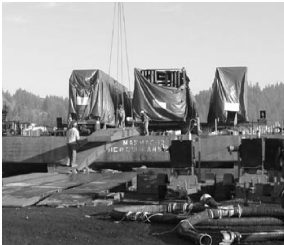
A crew prepares to unload heavy equipment for a new powerplant from the Foss barge Marmac-12 at Port Westward.
