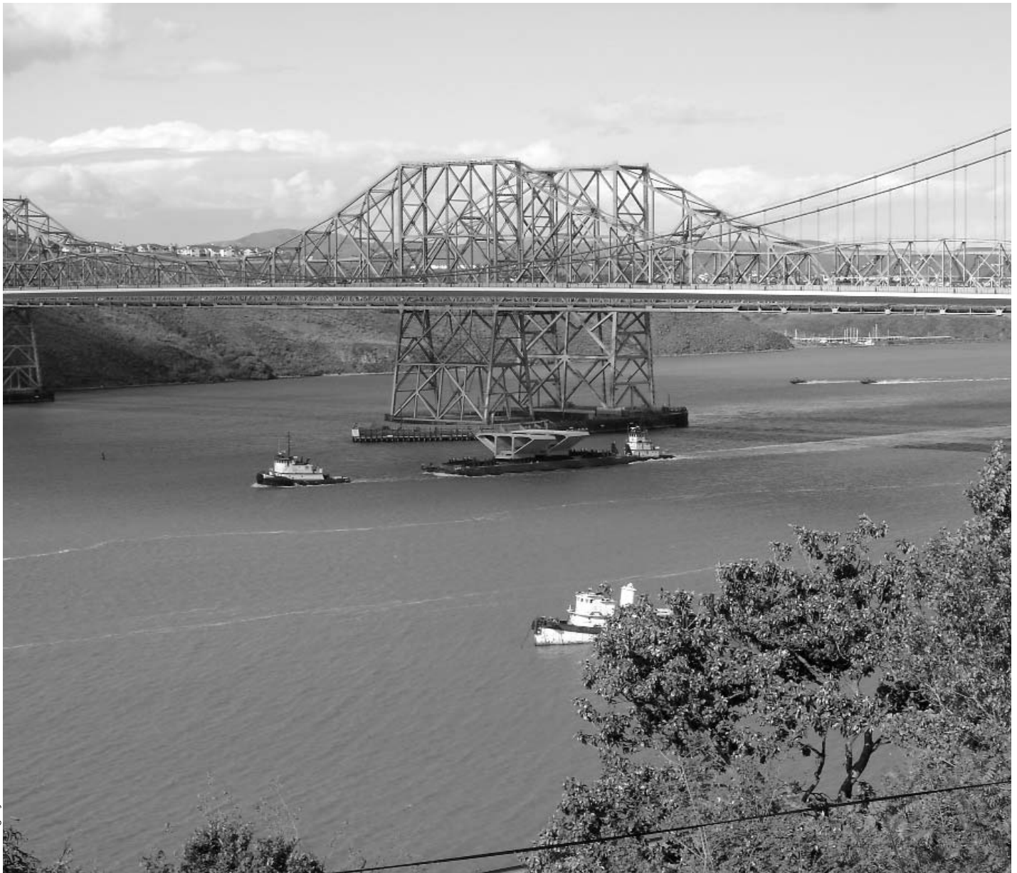
The Foss tugs Richard M, ahead, and Anna, pushing, move a bridge section under the Carquinez Strait Bridge.
