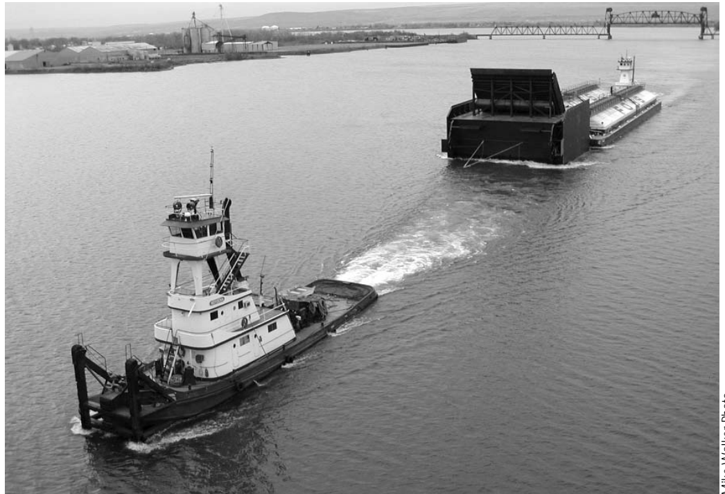
The Foss tug Noydena pulls the spillway weir up the Snake River toward Ice Harbor Dam, with the Clarkston pushing.
