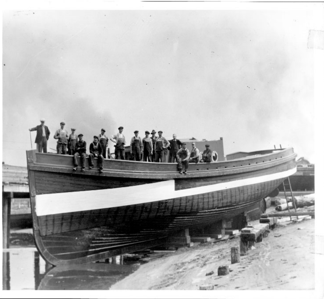
Shipwrights posed on the main deck as the completed hull of the Peter Foss was ready to be launched from Foss Marine Ways, Tacoma.
