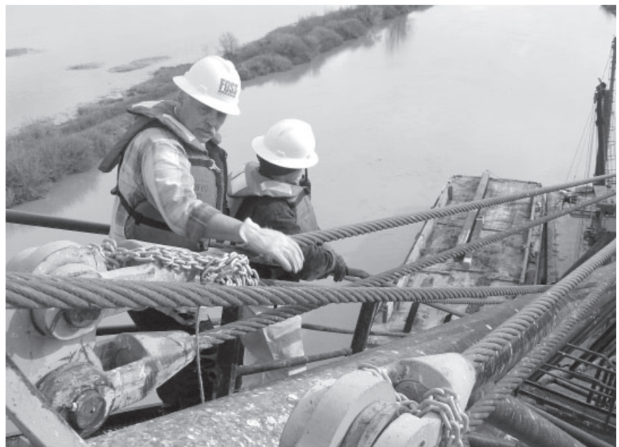
The boom of the old crane barge Monarch is inspected before the derelict is salvaged on the Sacramento River Delta.
