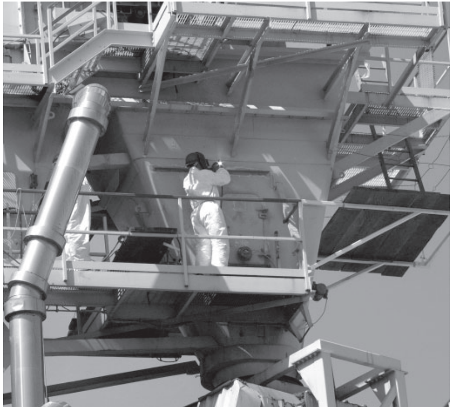
A welder works high in the superstructure of the Kivalina at Foss Shipyard, preparing the lightering barge for Foss' 15 th Season at Red Dog Mine.
