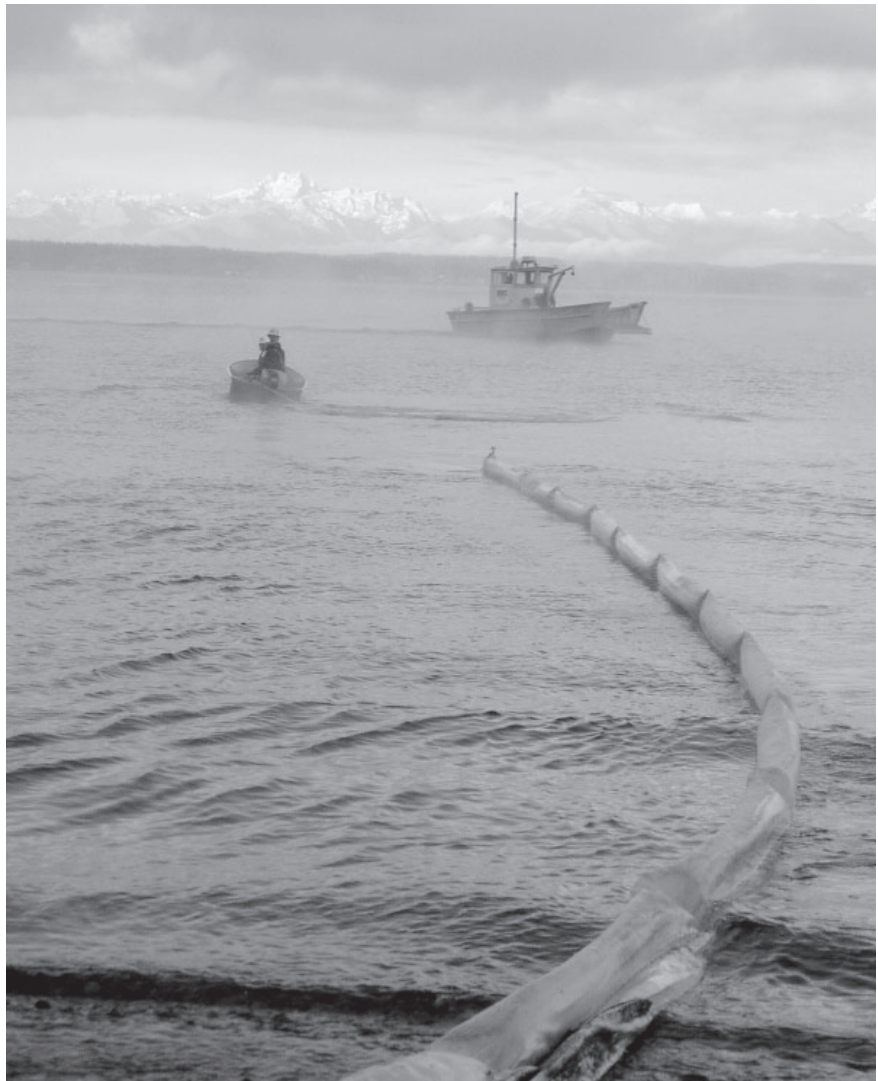
Containment booms were placed in the water at the Point Wells terminal following the spill.
