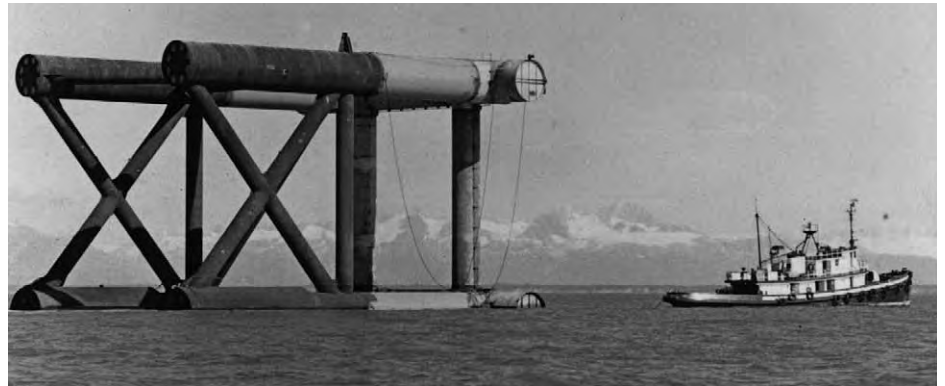
The Miki class tug Mary Foss arriving in Cook Inlet in 1964 with a drill jacket, towed in a horizontal position from San Francisco Bay. In order to right the jacket, the left side would be sunk to the sea floor, and the drilling platform would be mounted on top.
