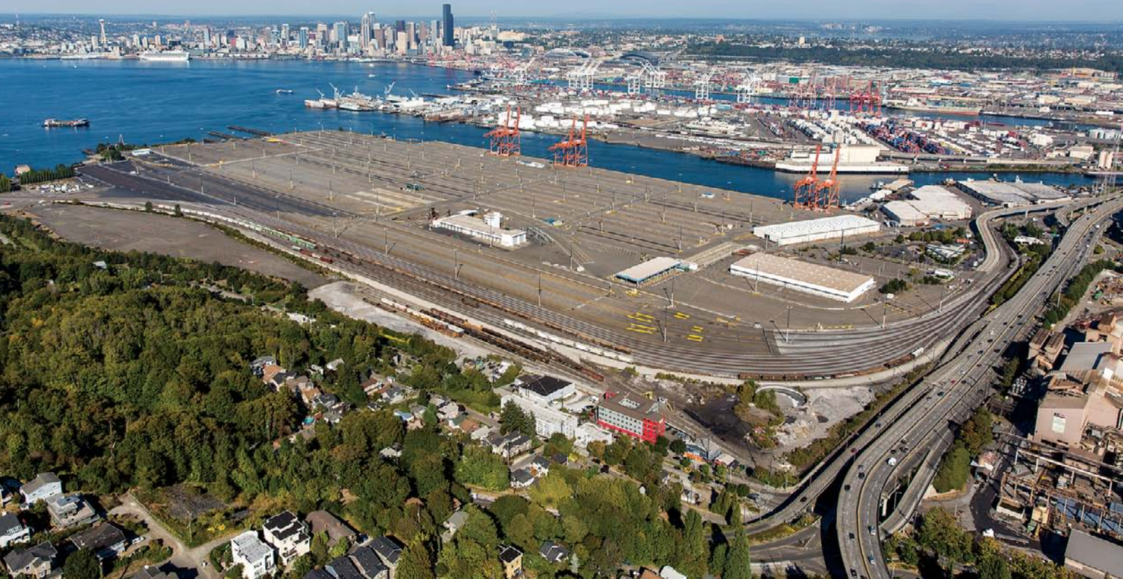
Foss is leasing about 50 acres of Terminal 5, which the port eventually hopes to develop into a state-of-the-art container terminal. Downtown Seattle is in the background.
