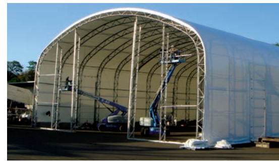
A fabric-covered, aluminum-framed building at Foss Shipyard in Seattle will house construction of two new fireboats for the Port of Long Beach.
