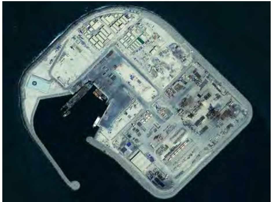
Aerial photos shows barge Mariner in its berth at South Island.
