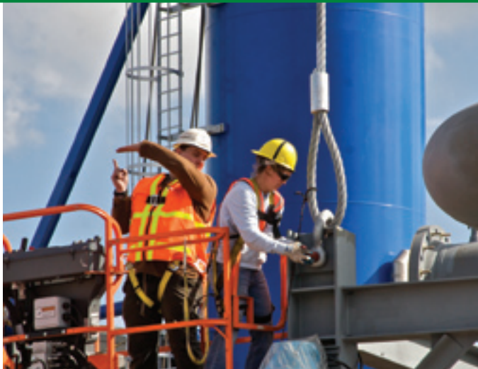
A longshoreman fixes a shackle to a module before it is lifted onto a Foss barge at the Port of Vancouver.
