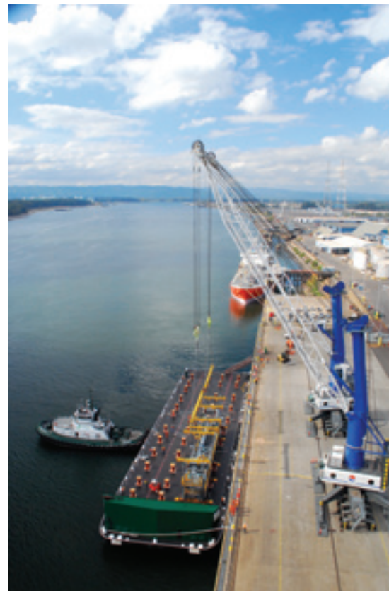
The Pacific Escort stands by as two big Liebherr cranes lift the first module onto the specialized barge Foss 286-3.
