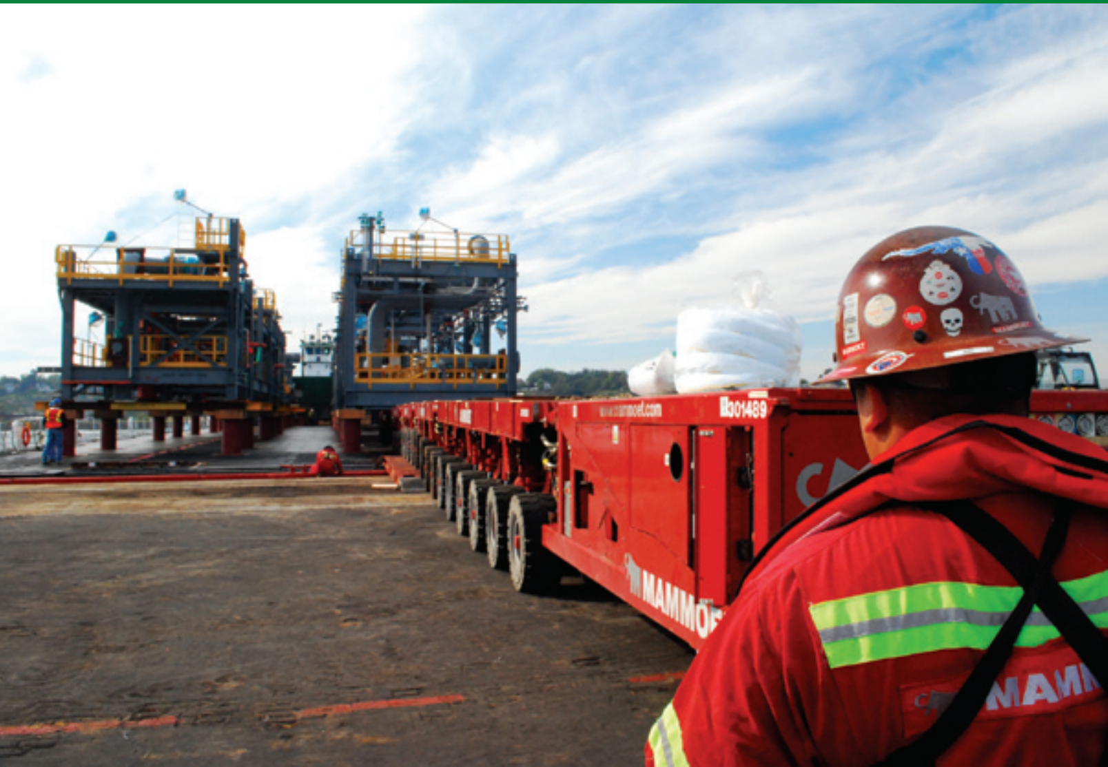
An employee of heavy-lift company Mammoet is controlling a self-propelled modular transporter (SPMT) to offload modules at the Port of Lewiston.
