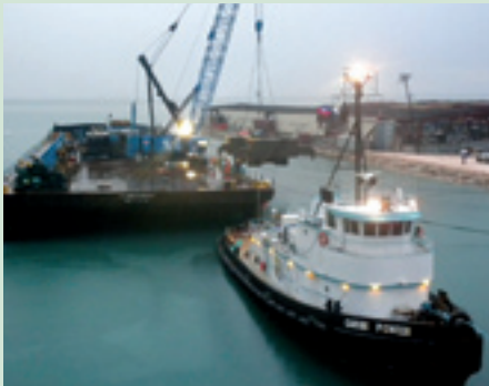
The Caribe Pioneer stands by as a lower section of the crane is hoisted onto the barge Columbia Boston .
