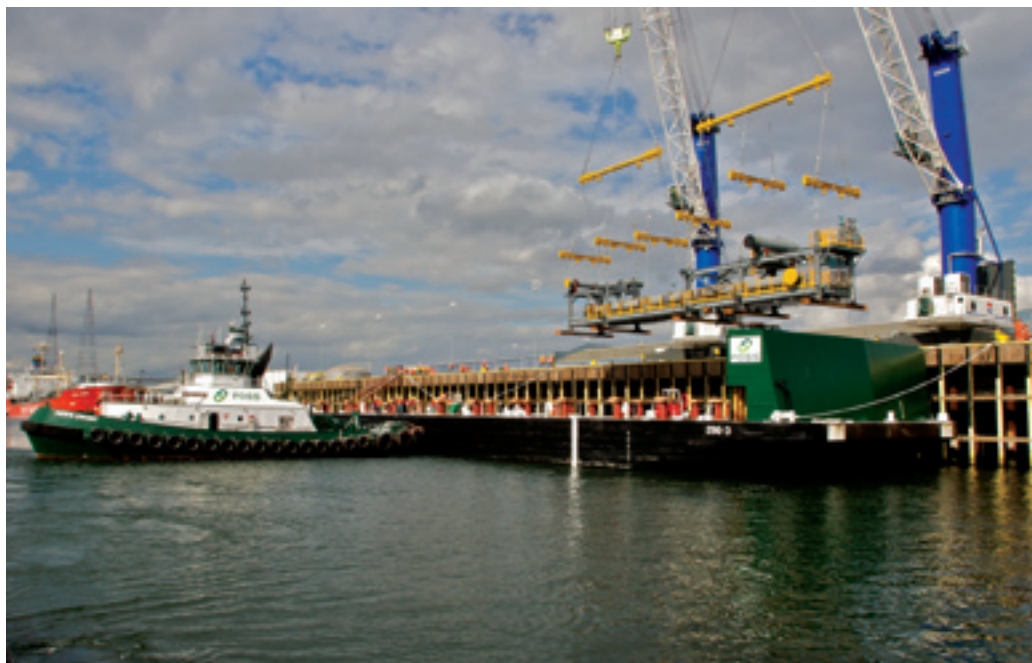
The first module is loaded on the Foss barge 286-3 at the Port of Vancouver, Wash., on Oct. 8.
