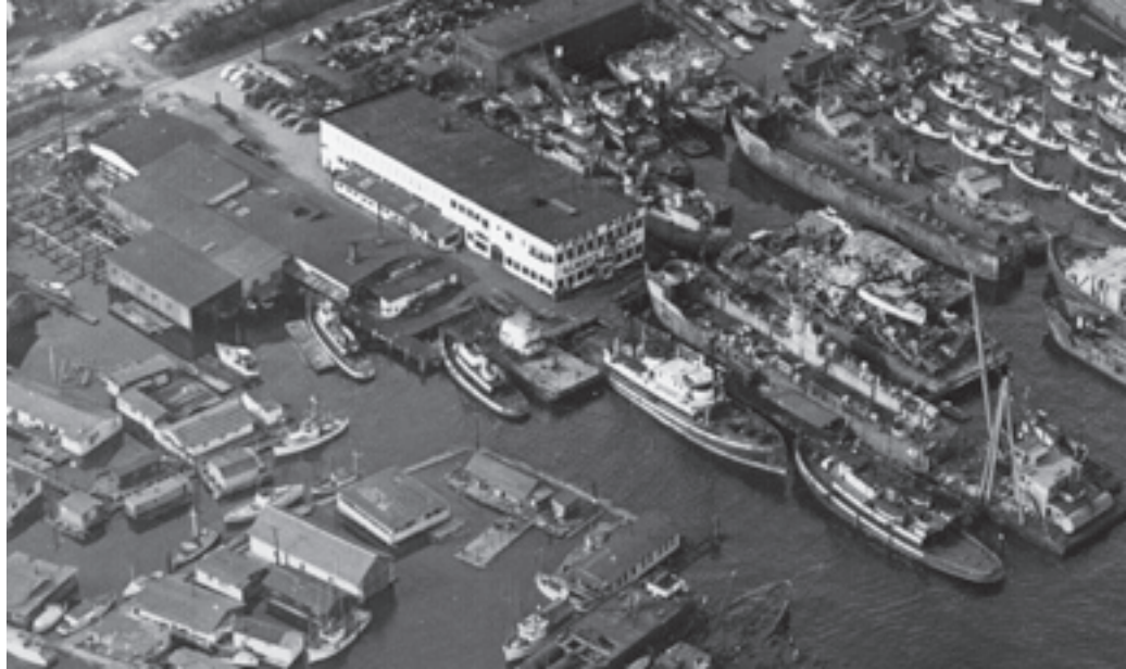
A 1949 photo of the current Foss property on Ewing St. The carpenter shop and other repair facilities are located in the buildings to the left of the white administration building. The area where the current shipyard and terminal are located was used as moorage for war surplus vessels purchased by the Foss family, as well as barge storage and public marinas. The building currently housing the Purchasing and Billing Department is also visible in its current location, just to the right of the back of the administration building.
