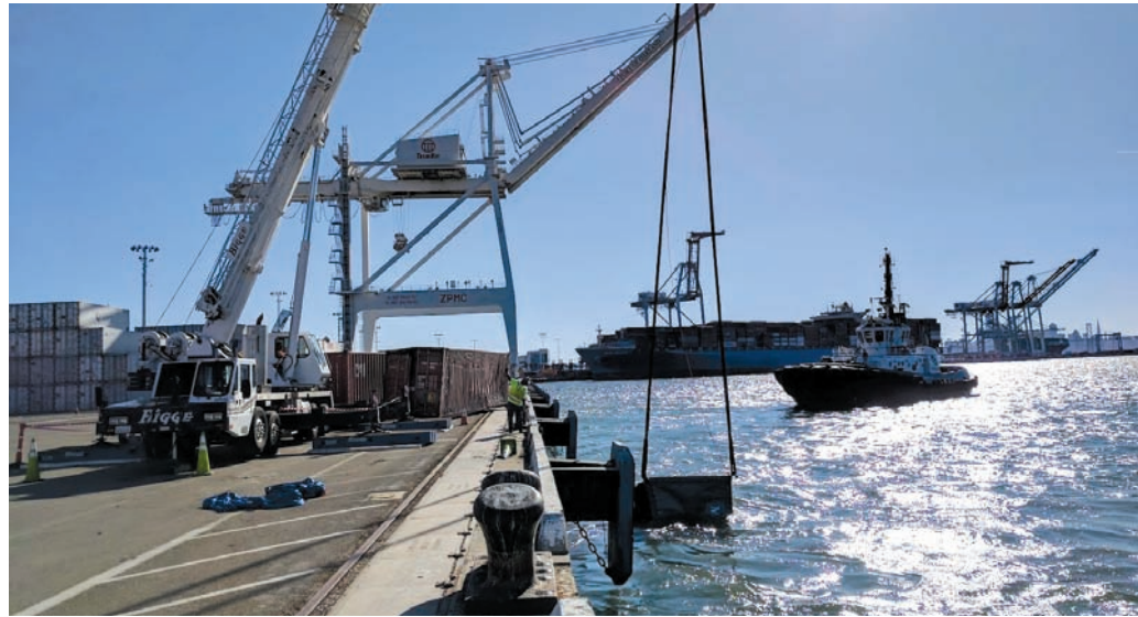
The tug America stands by as a dockside crane lifts a sunken container onto the pier.
